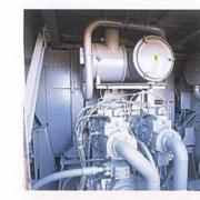
■ Engine-pump bulkhead is provided to between the engine and pump.
