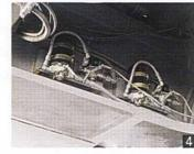
4 The air drier eliminates moisture inside the air piping
